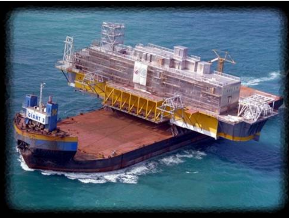
Visund LQ & Utility Section
