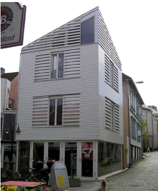
Steinkargaten 21 – a small commercial building in the historical core of the city
